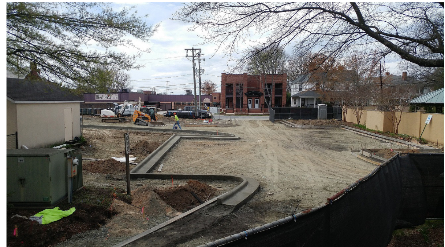
Completed concrete curbs framing the new parking lot
