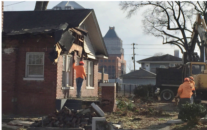
Demolition of residential buildings on campus
