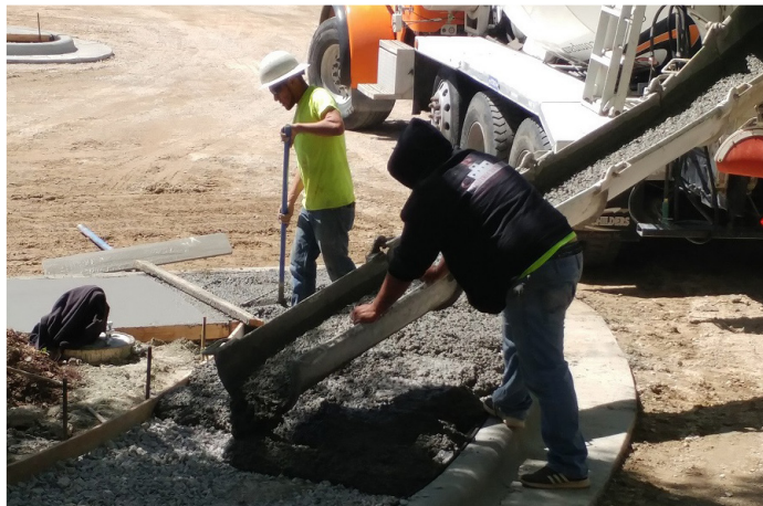
Laying new concrete curbs in parking lot
