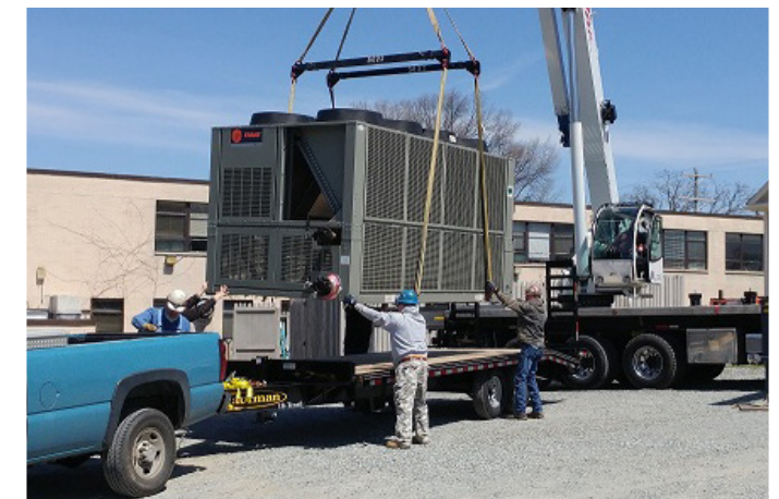
Moving chiller to clear the way for work to begin in Phase II on the covered terrace adjacent to the Haywood Duke Room
