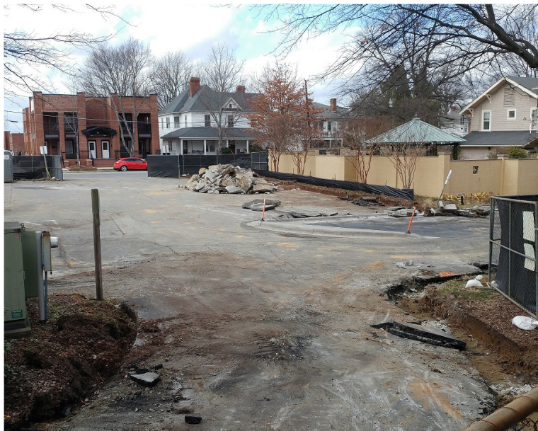
Demolition of the parking area behind the Fisher House
